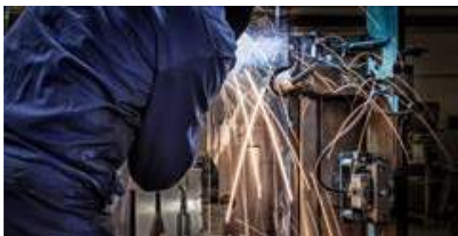
Welding of frame
