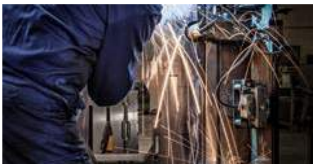
Welding of frame
